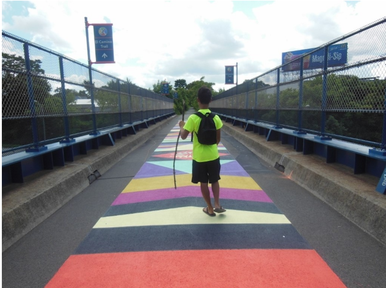
Bridge on the El Camino Trail
